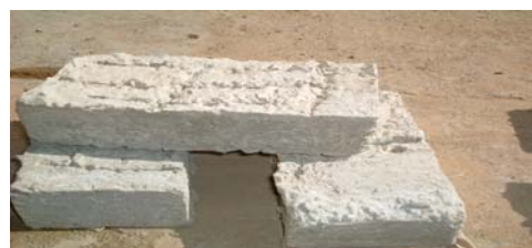
Figure 1: Ordinary concrete substratum
